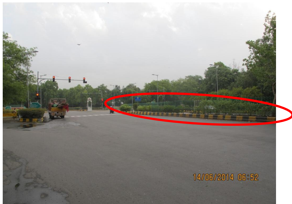
Figure 2.4: Overgrown Suburbs at the Median Portion on the Aurobindo Marg Approach obscuring the visibility of the traffic emanating from Prithviraj Road Approach until it reaches the mouth of the intersection (a) (i.e. Oblique Angle of meeting of the Prithviraj Road Approach)
